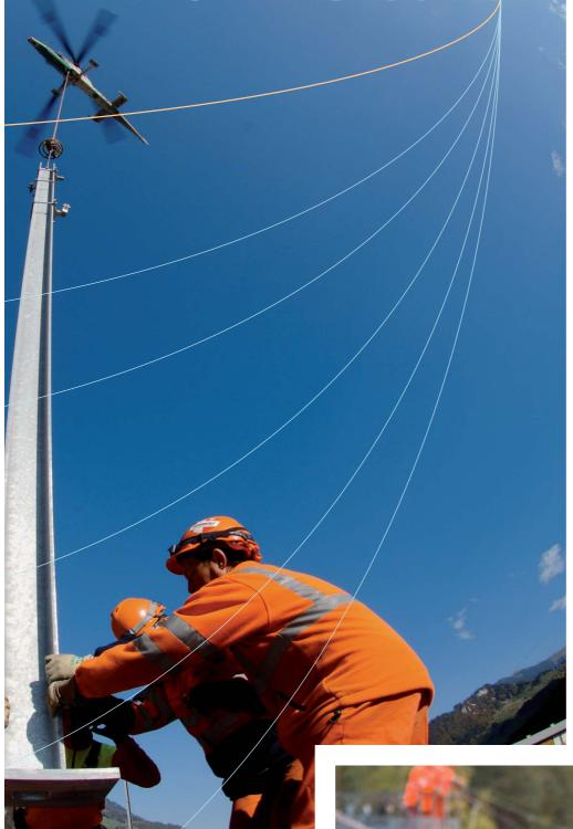
In principle we do not want to disturb railway operation. Where possible our components arrive preassembled at the construction site and are presorted in the right order. If the environment permits we erect fully assembled masts using a helicopter. For the rest we rely on our planning teams.
