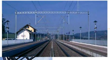
Over recent years, overhead contact line systems FL 200 and FL 260 have developed to become a standard and have recently also found approval abroad. Characterising this overhead contact line system is the small number of components, a suitable planning tool and its resistance to corrosion.
